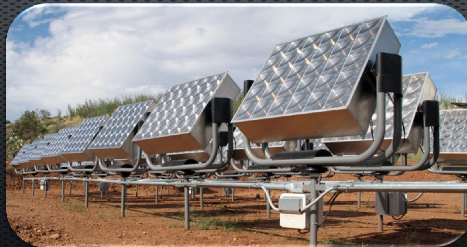
Typical HCPV (High Concentrated Photovoltaic) Array
